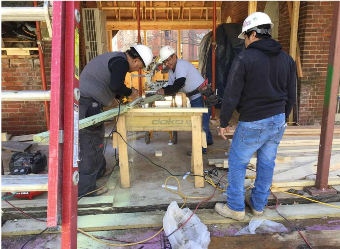
Six carpenters are at work.
