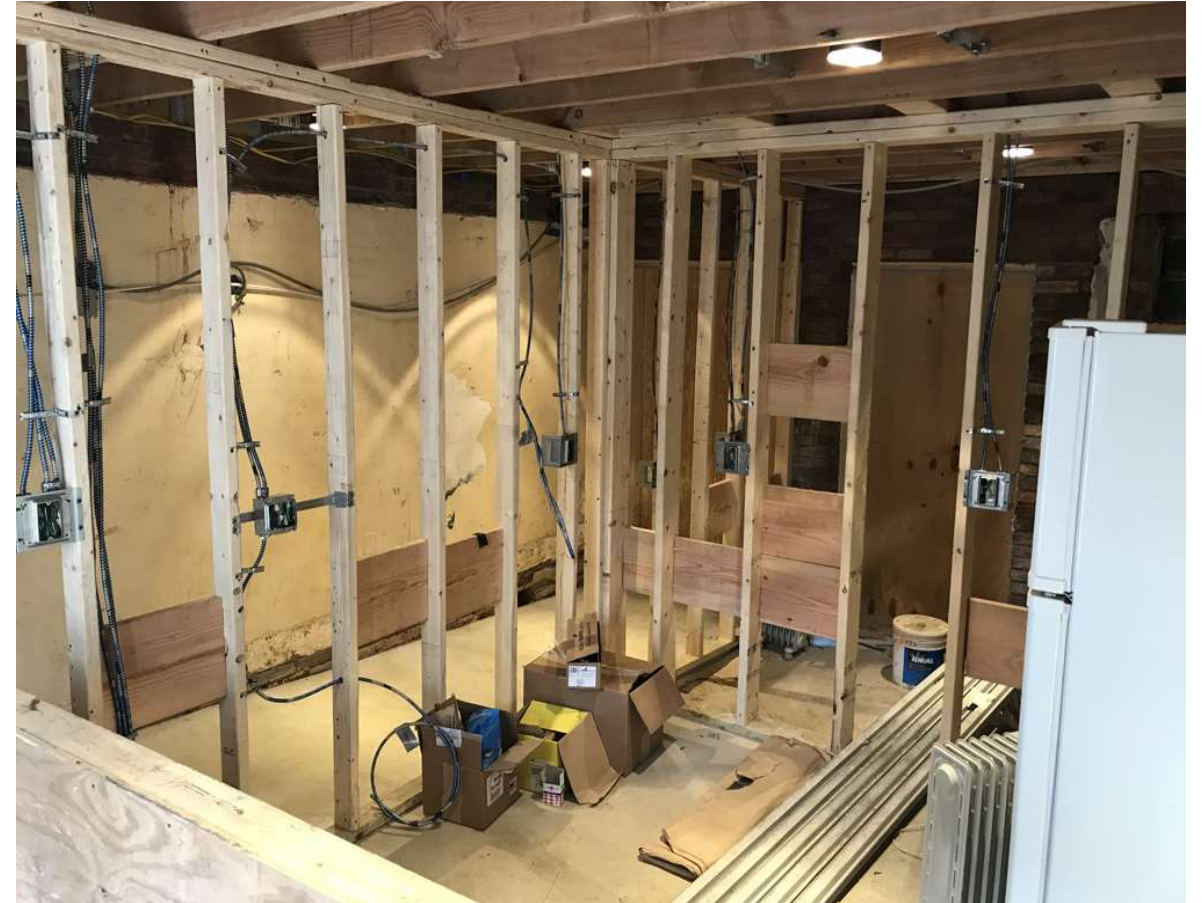
Electricians continue to work on the Carriage House kitchenette/bathroom hallway.
