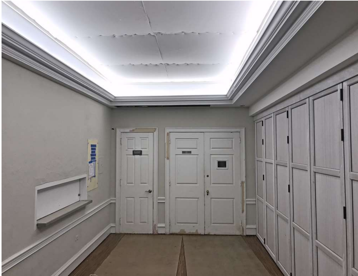
The ceiling installers make some progress.
