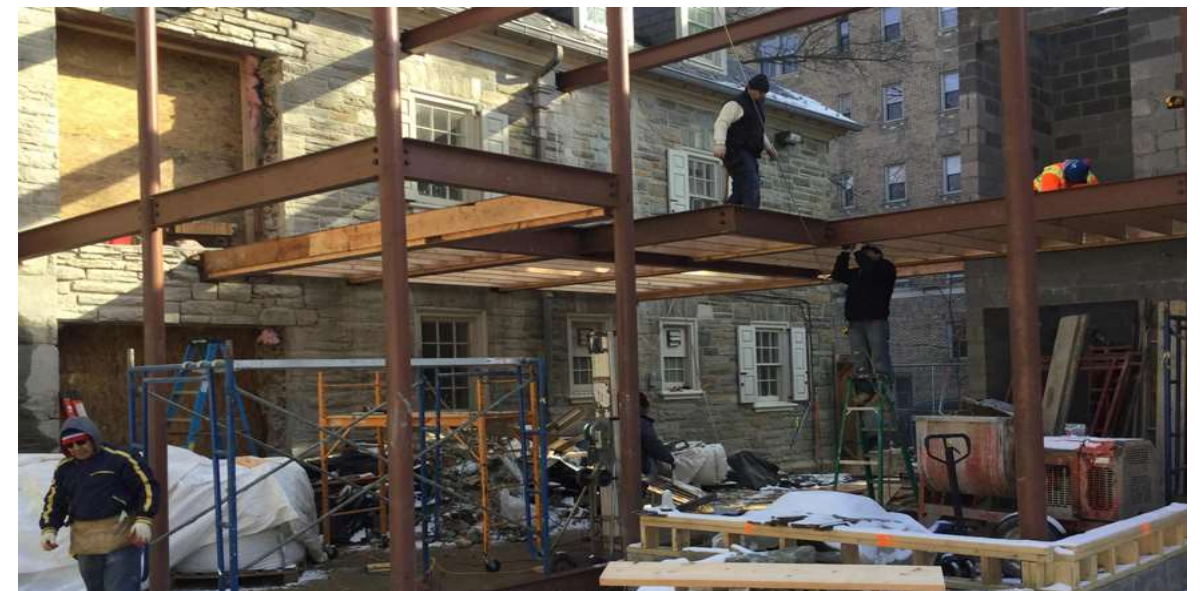
Others are adding to the framing for the HVAC compressors on the roof and the framing for the upper level Lobby floor.
