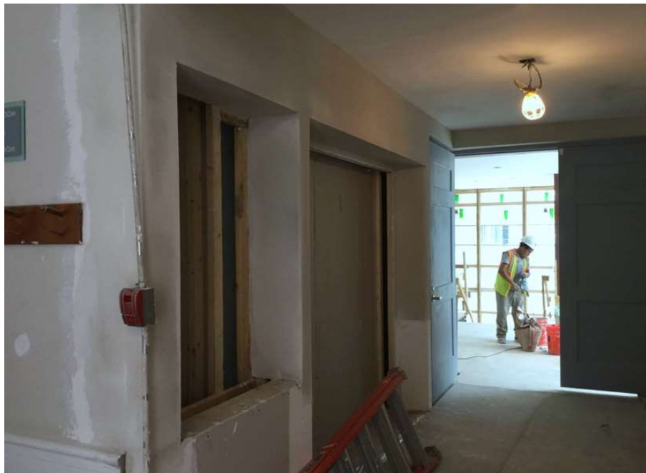
Three plasterers put a finish coat on the Parlor hallway.
