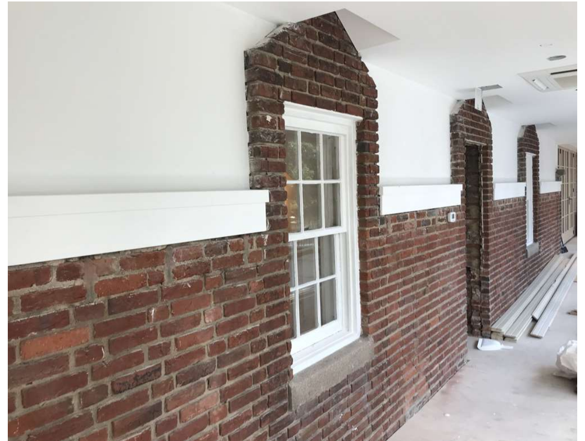
A painter spruces up the old Carriage House windows.
