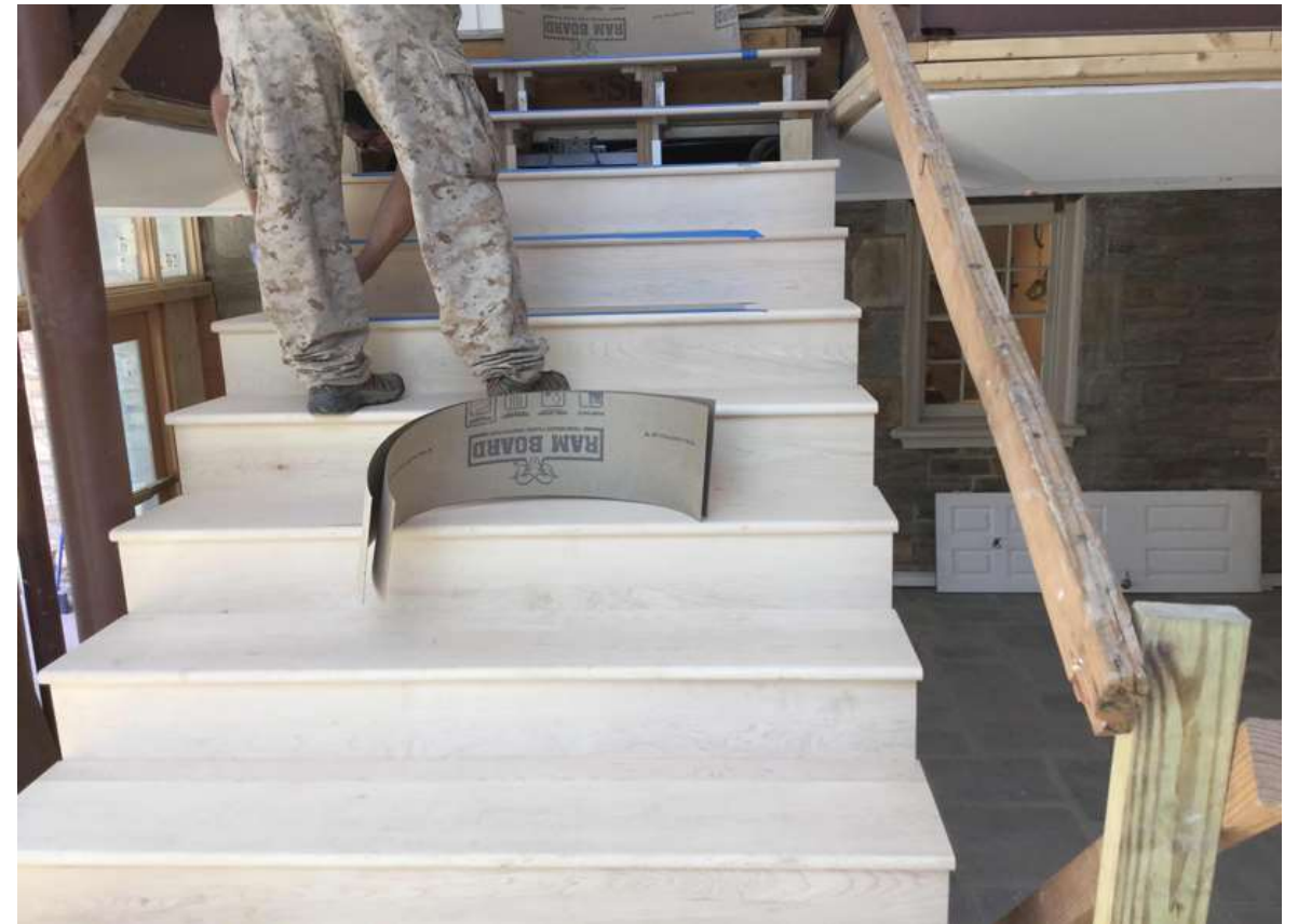
Three stairmasters work on the Lobby stairs.
