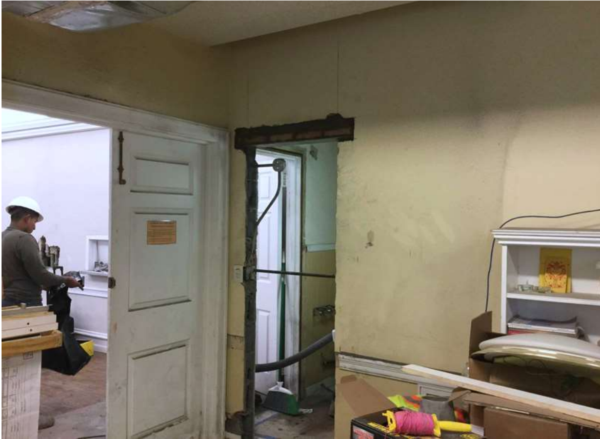
The tiny Assembly Room bathroom acquires a new door opening
