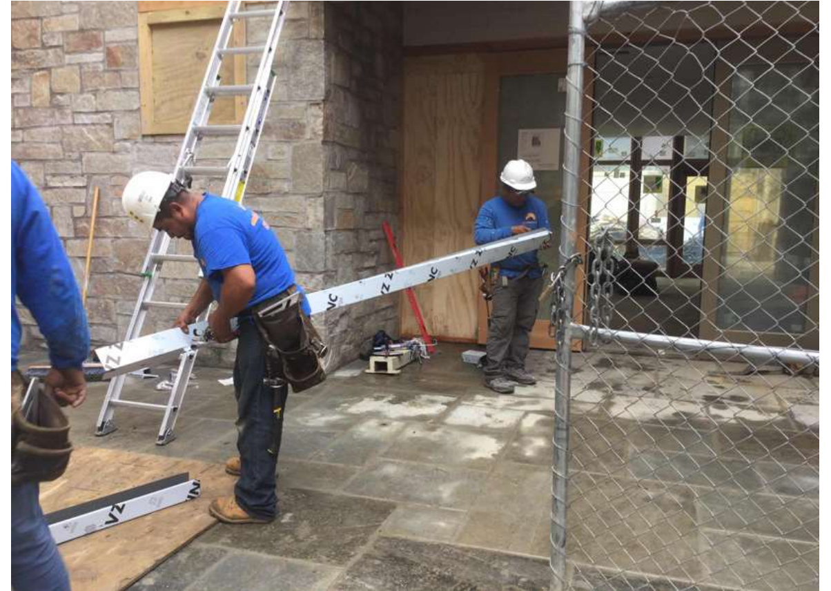
Four roofers install gutters and Lobby entrance roof panels.
