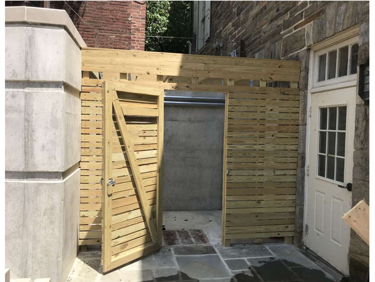
A reconfigured, slightly less fortresslike trash alcove wall and gate.
