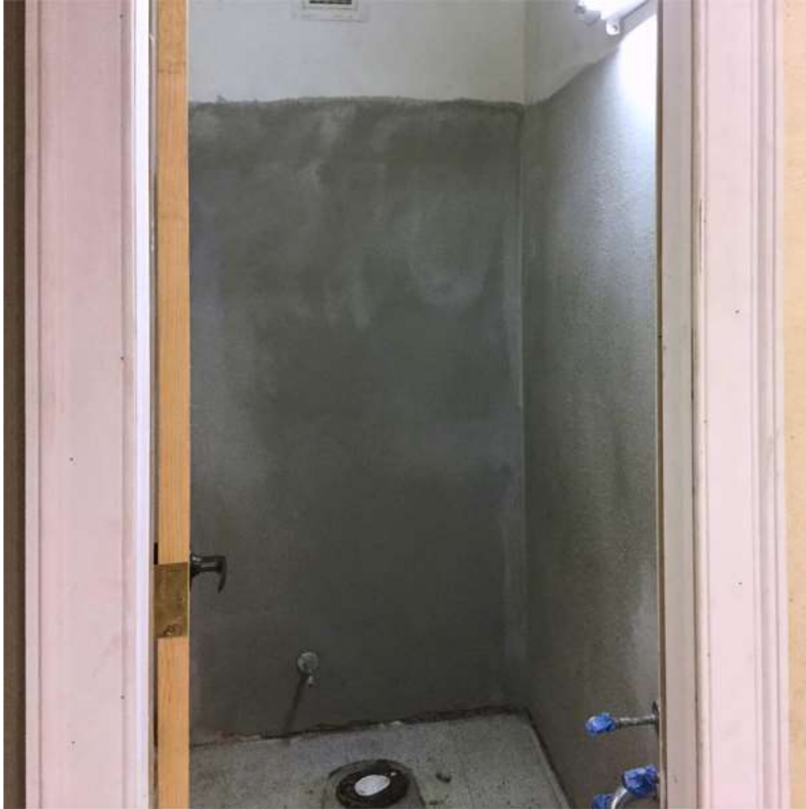
Plasterers conceal the walls in the small Assembly Room bathroom.
