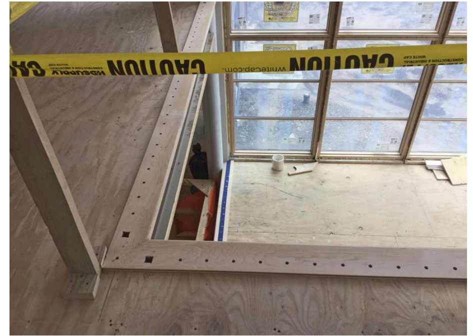
Douglas and Mario continue to drill holes for stair railings.
