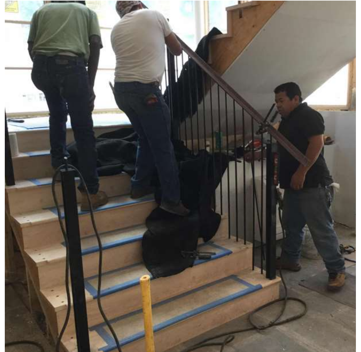
The ironworkers continue the railings down the stairs.
