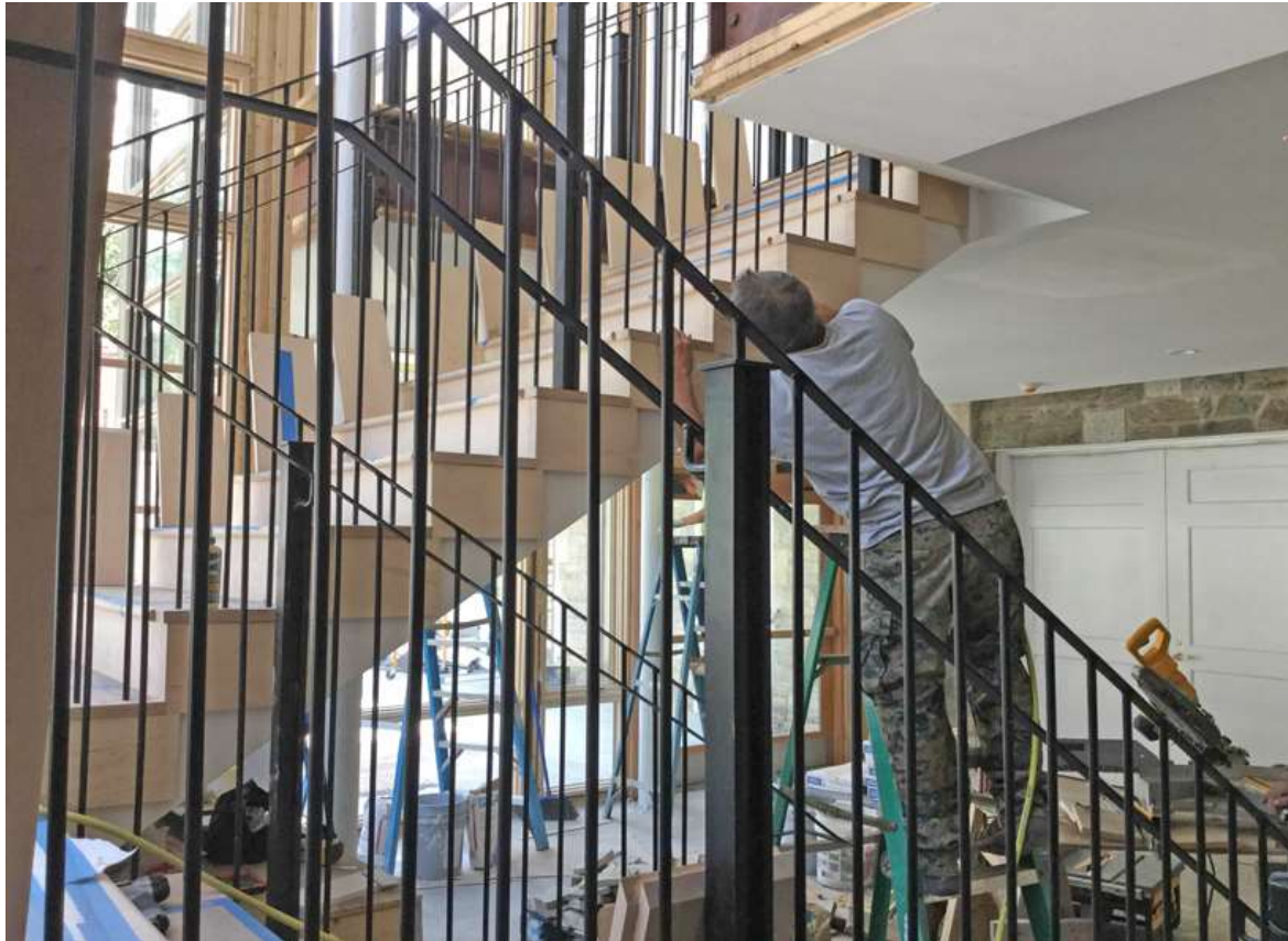
Two stair installers work on stair returns.
