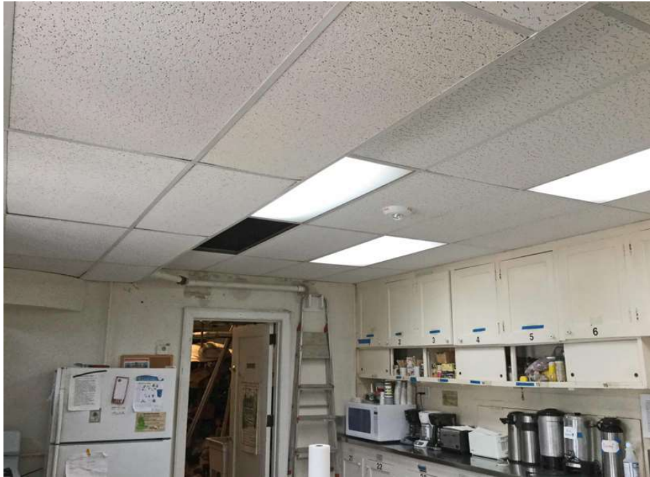
Mario and Douglas reinstall the Kitchen ceiling.
